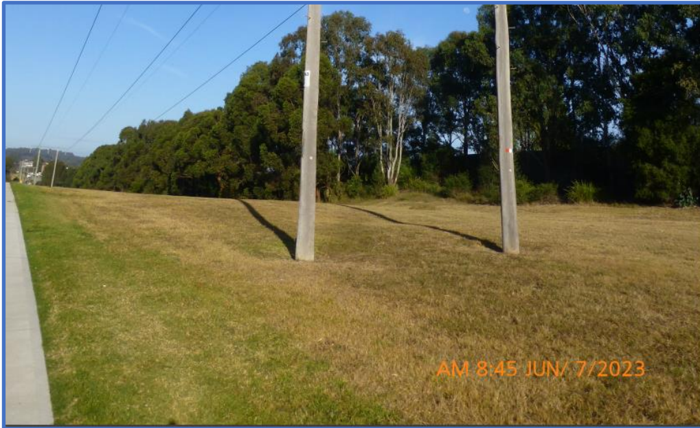
Figure 18: Ground surrounding Pole 3 to be replaced
