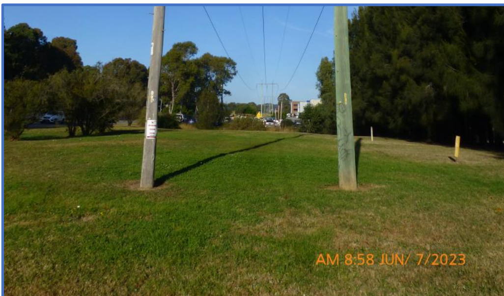
Figure 19: Ground surrounding Pole 5 to be replaced
