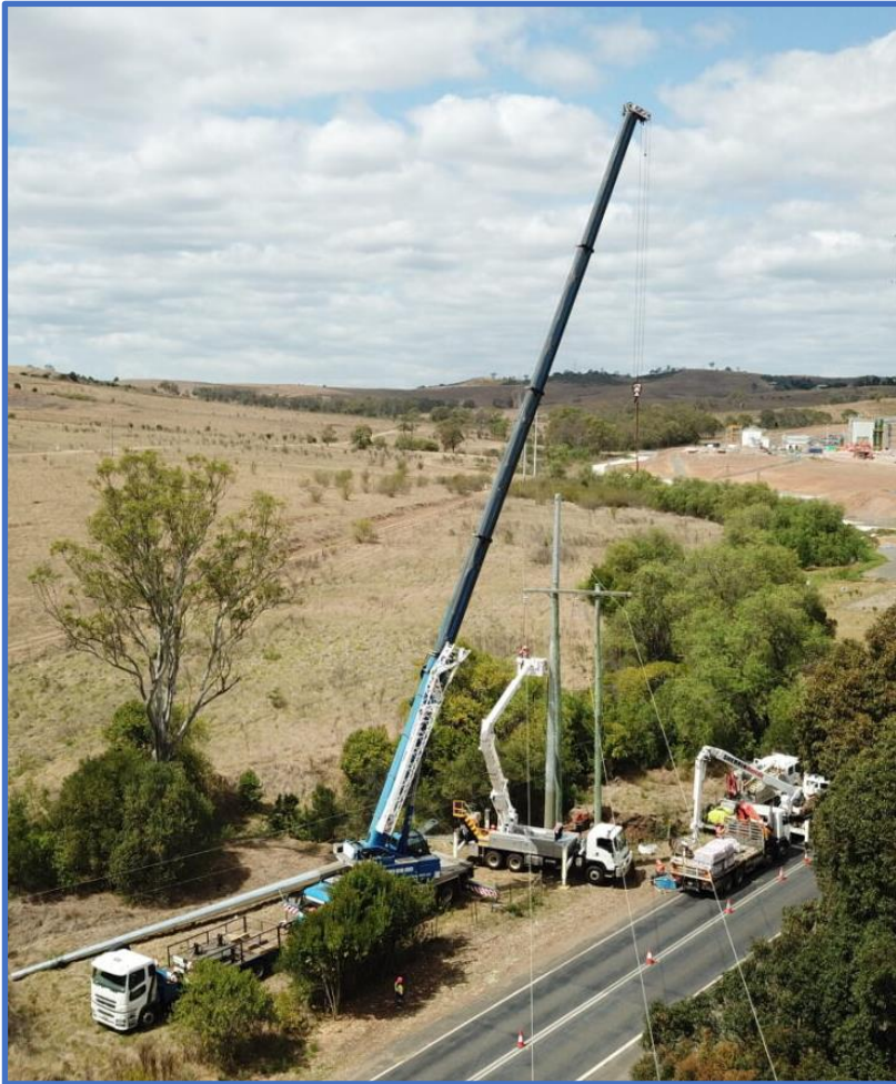
Figure 12: Example of pole replacement works
