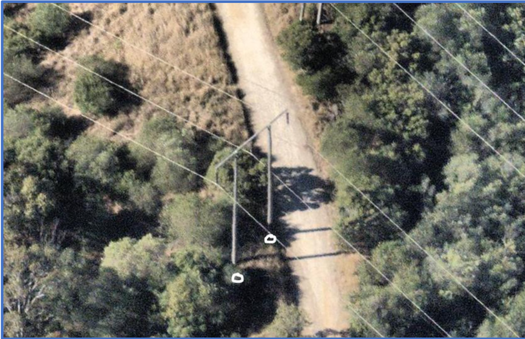
Figure 22: Satellite image showing Pole 15, with markup indicating approximate proposed position of replacement poles
