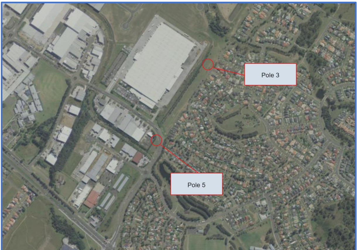
Figure 26: Satellite image of vicinity of Section 1 of proposed works
