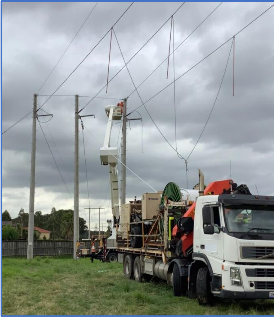
Figure 14: Example of conductor replacement process
