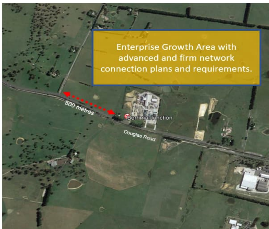
Figure 4 – Aerial view of the Berrima Junction Enterprise Growth Area including the existing Zone Substation
