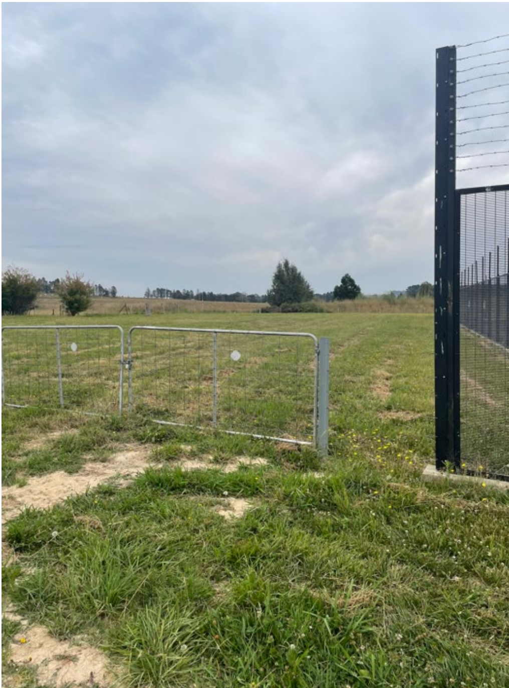
Plate 2. Current Berrima Junction Zone Substation
