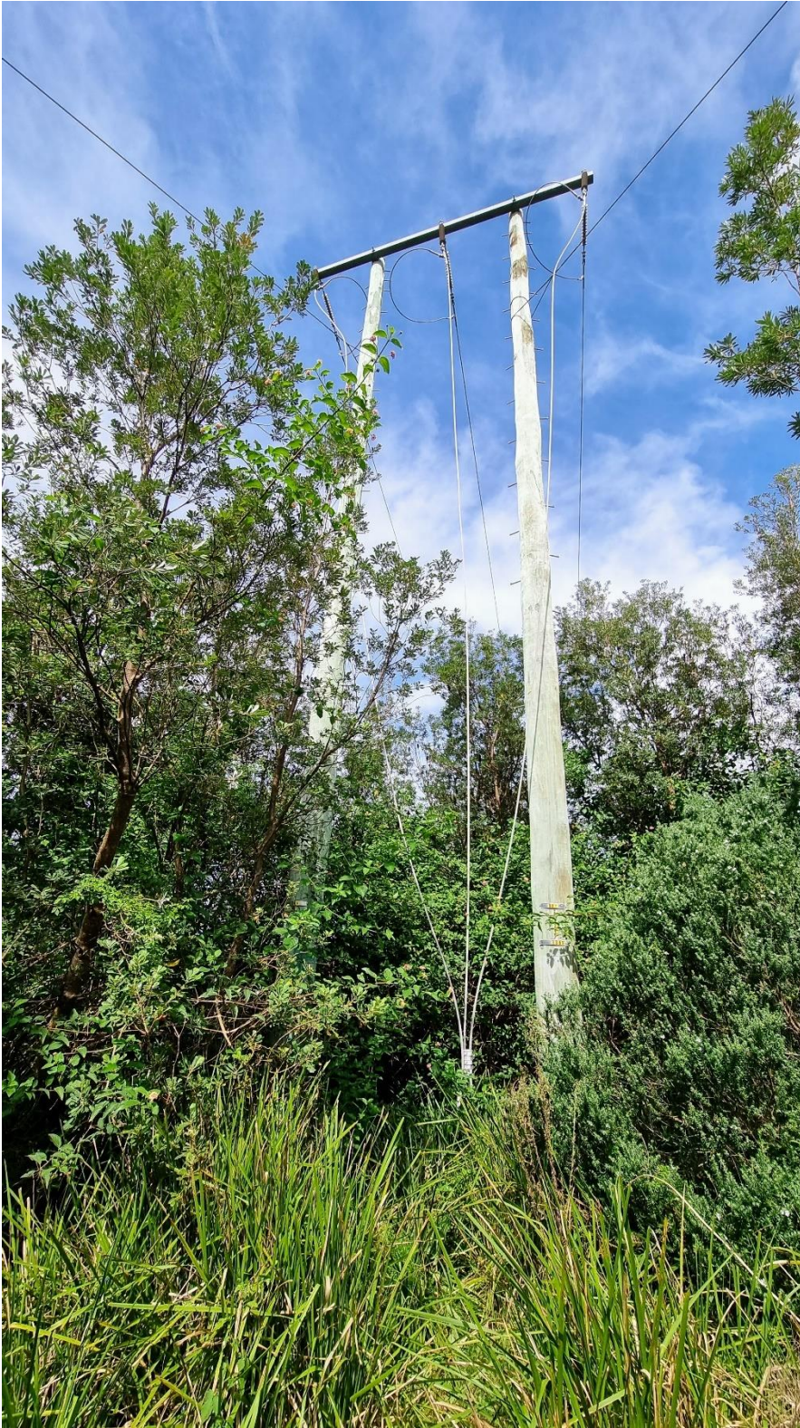
Photograph 7.2 H Pole structure (poles 878259 and 878260) on southern end of Picnic Island
