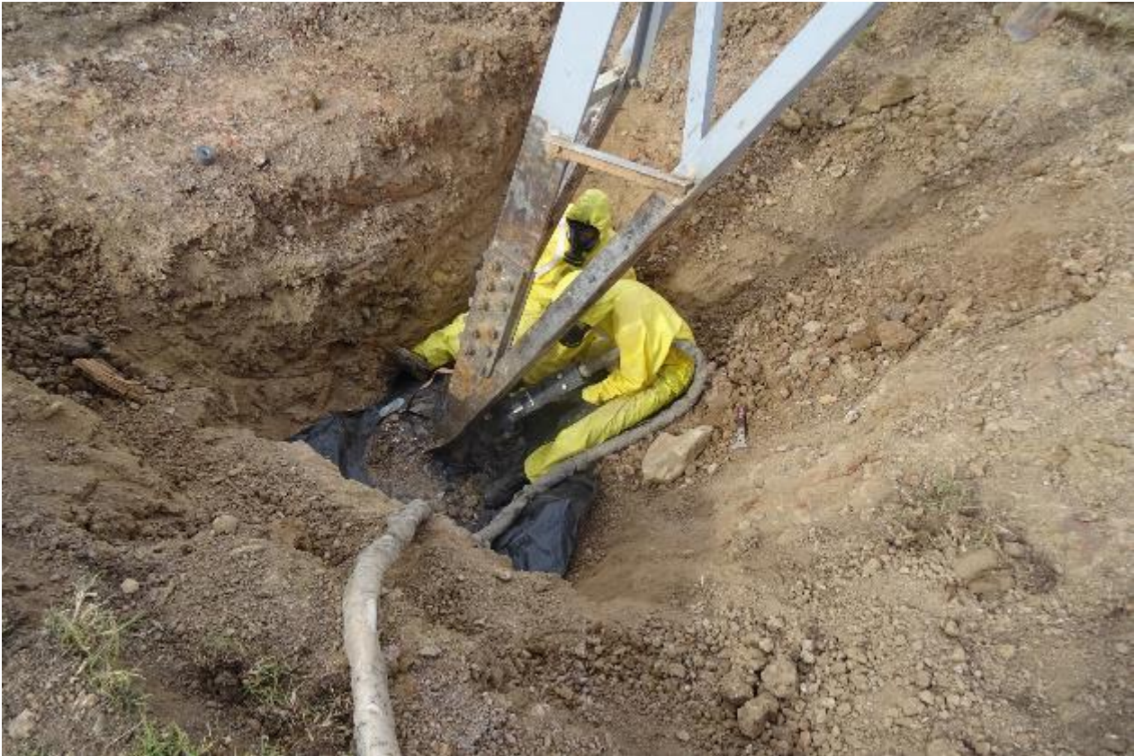
Figure 2 Example of excavated grillage foundation
